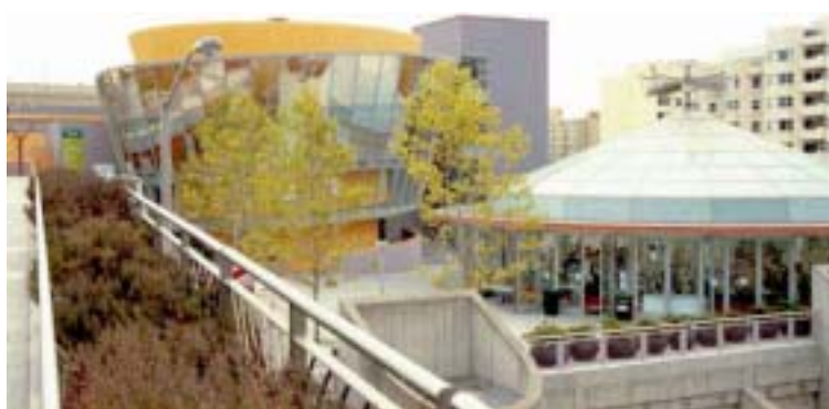
This view of the Moscone Center, the Zeum Childrens Museum, and the Loof Carousel illustrates the unique design of the facility, which will soon be home to a 675-kW solar electric system.
