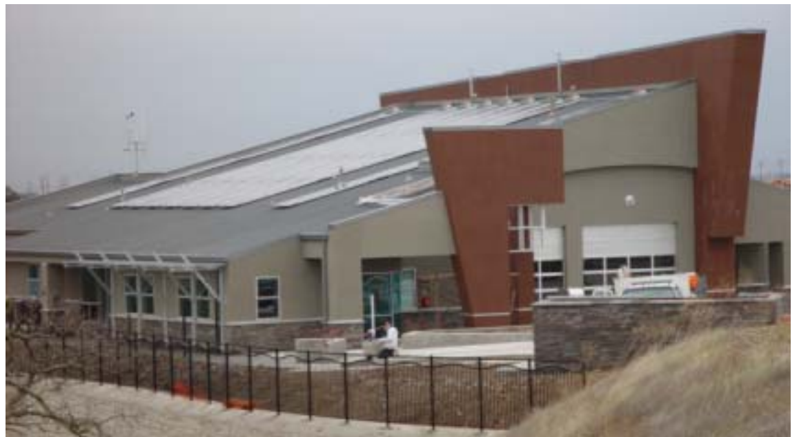
Roseville's new fire station features an 18.2-kW solar electric system, just one of many PV systems in the city.
