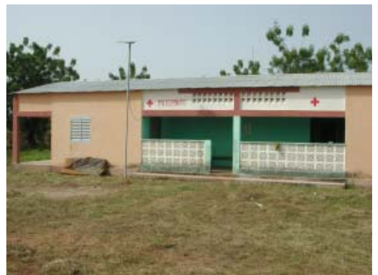
A solar electric system provided by the ACCESS program provides electricity to this maternity ward in Ourikila, Mali.
