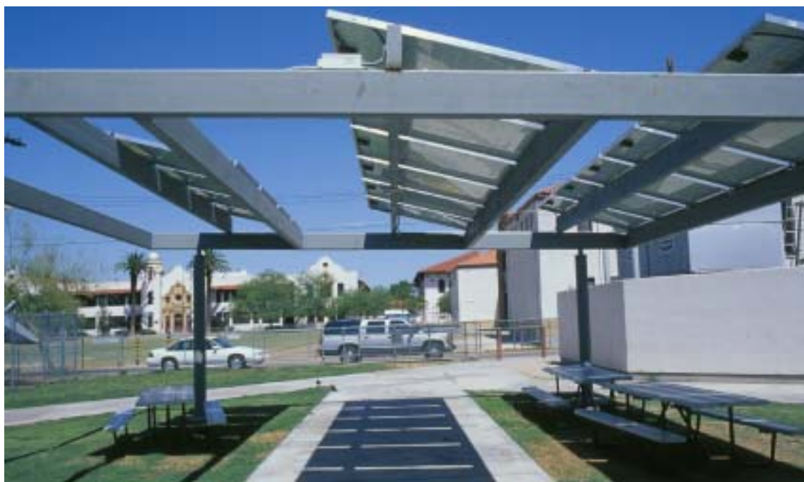
Teachers at Safford Middle School often use this porch, shaded by a 4.8-kW solar electric power system, to conduct class, enabling students to experience the workings of a solar electric power system up close.
