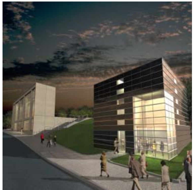
Solar electric modules will be integrated into the glass façades on the Millennium Park's energy-efficient, black-glazed cube-style pavilions.
