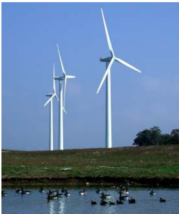
These three wind turbines, located in Somerset County, Pennsylvania, annually supply 9,375 megawatt-hours of green power to American National Wind Power and Green Mountain Energy customers.
