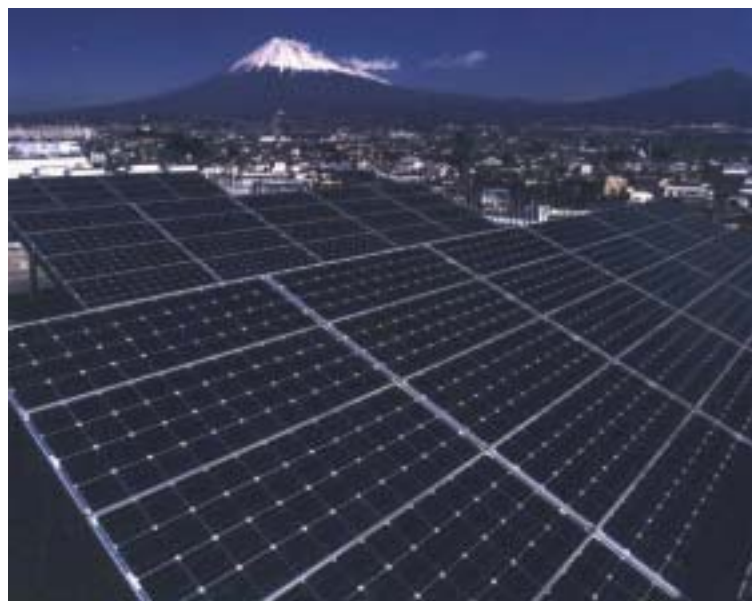
TEPCO's offices in the shadow of Mt. Fuji feature solar electric power.
